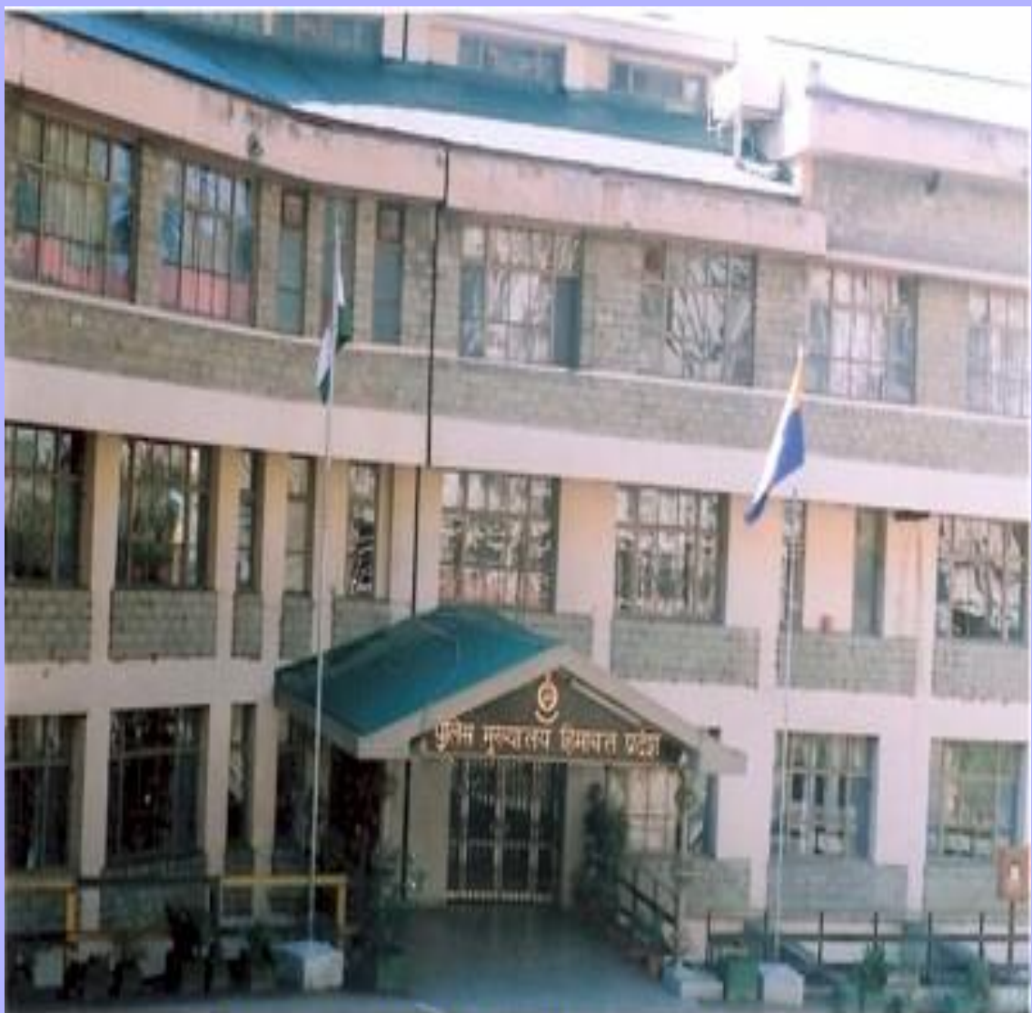
Front view of HP Police Headquarters Shimla
